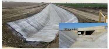
Second Phase of Firebaugh Canal's 1st Lift Canal Lining Project included lining some 2 miles of canal for improved efficiency, maintenance and delivery.
