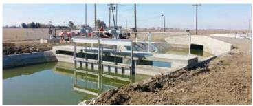
The project also included construction of a new automated check structure that will be operated through the District's SCADA system.
