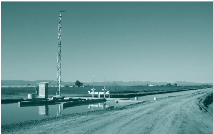
Canal improvements include the installation of weirs and SCADA systems to reduce operational spill and enhance automation.
