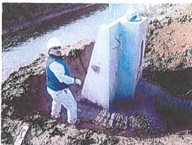
Figure 15. Installation of GCID metergate
