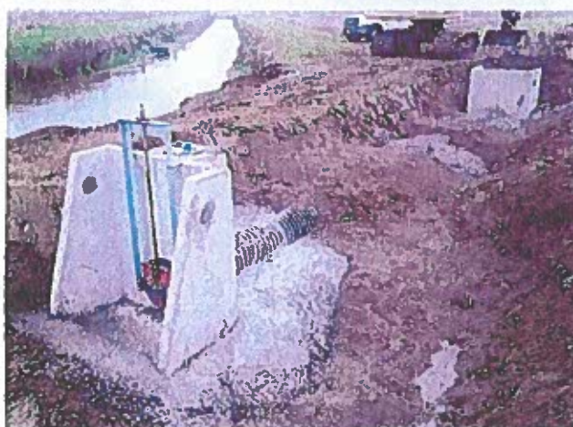
Figure 16. Final concrete for GCID metergate, showing downstream pre-cast outlet box
