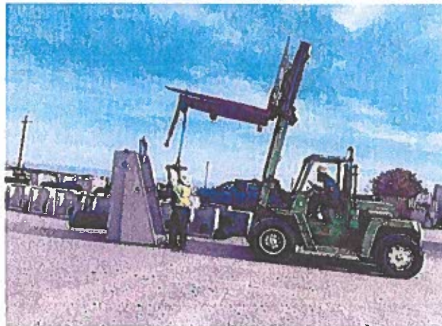
Figure 14. Pre-cast metergate ready for transport
