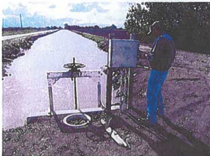
Figure 12. Large diameter stilling well, with cover to minimize having it fill with dirt from the road. Strong concrete, with the rim of the stilling well at the same elevation as the bulkhead top.
