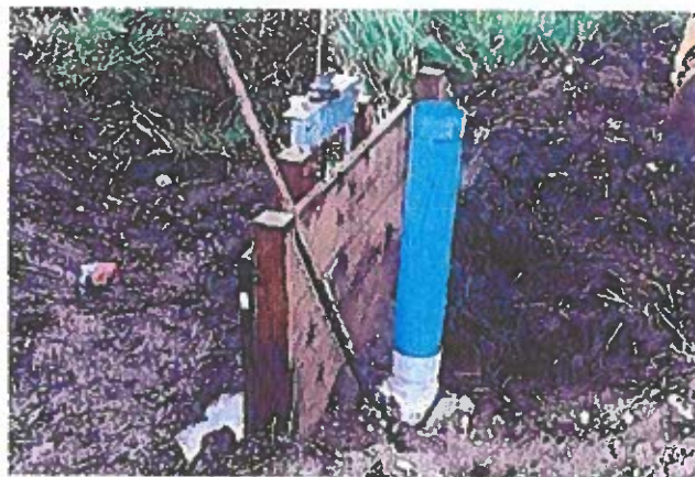
Figure 8. Stilling well installed on an existing discharge pipe. It is constructed of PVC pipe that is too thin for long life, but it serves as an example of the correct diameter, position, and height.
