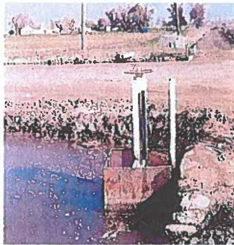
Figure 11. Correct height of stilling well to match top of gate frame. However, the diameter is too small. Steel pipe material is good
