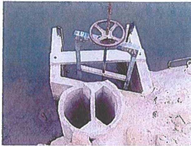
Figure 9. An old type of dual-stilling well commonly found in Central California irrigation districts. One stilling well was connected to the canal, and the second was directly over the discharge pipe. The idea of measuring down into both stilling wells from the same center point was good, but the top of the stilling well was so close to the ground surface that road maintenance quickly filled these stilling wells with dirt. Also, the side connection between the canal stilling well and the canal itself was too difficult to clean.
